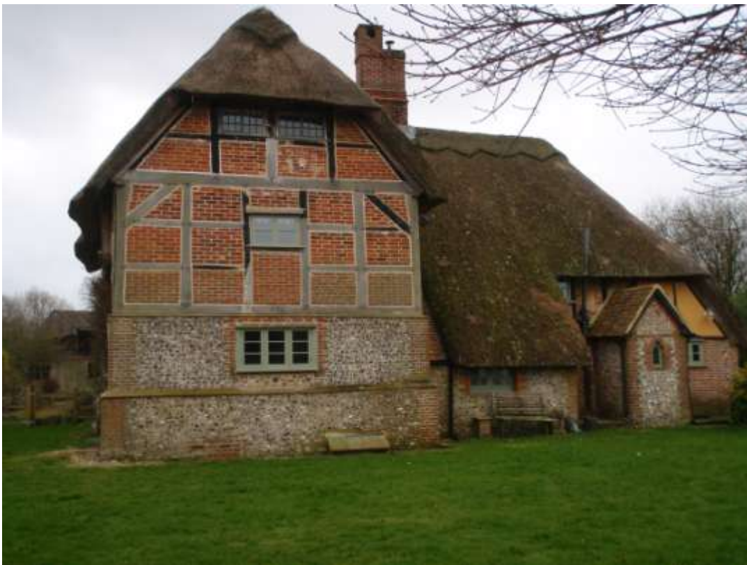
Plate 6. View of Site (looking south)
